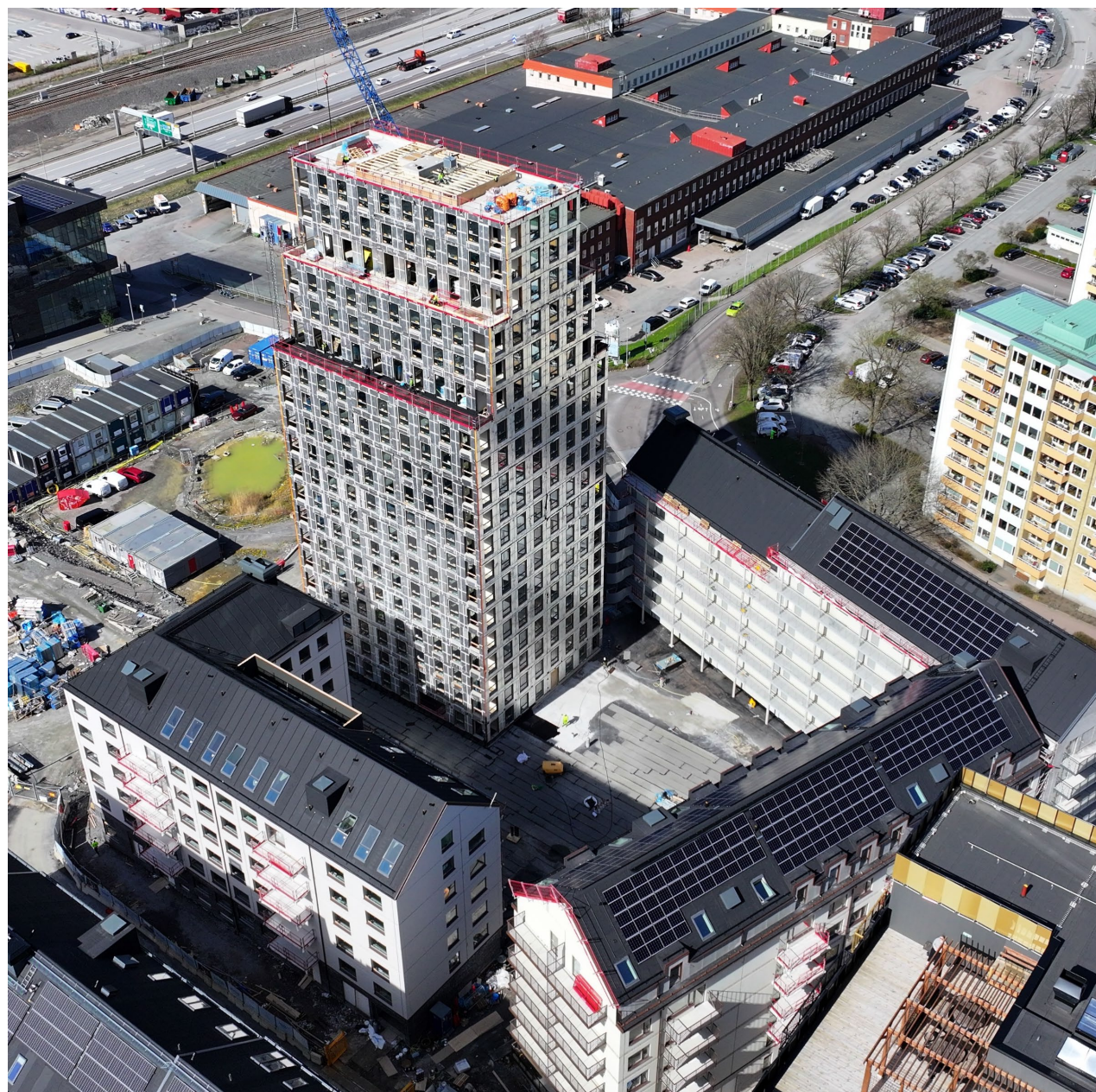
Kv. 6, Kallebäcks Terrasser, Gothenburg
