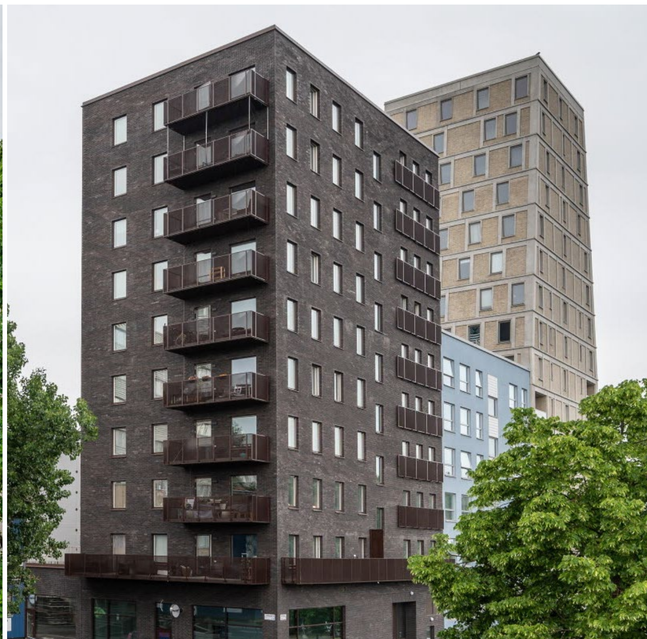
Umami Park, phase 1A, Sundbyberg, 38 rental apts.
