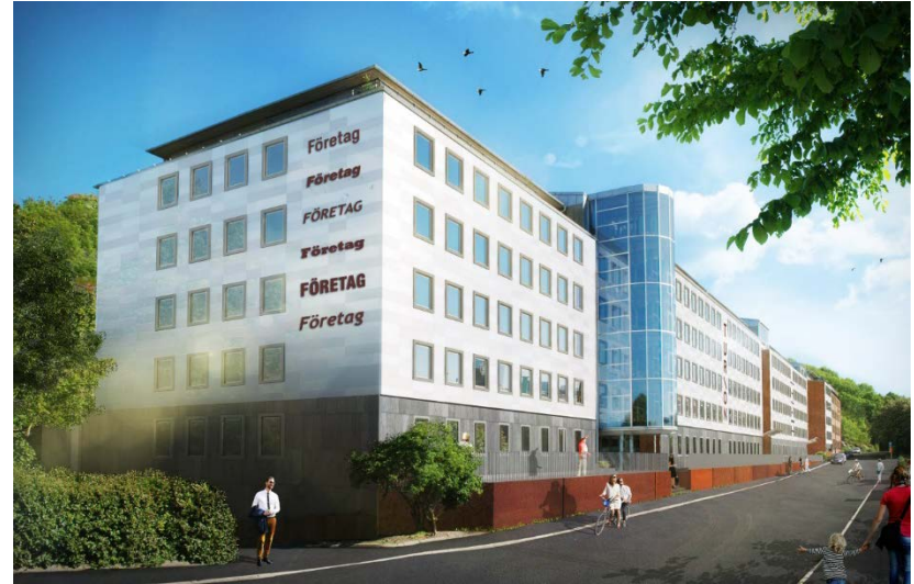
TURION IN GÅRDA: ONGOING UP-GRADING AND MODERNIZATION, INCL. ENERGY SAVING PROJECT
